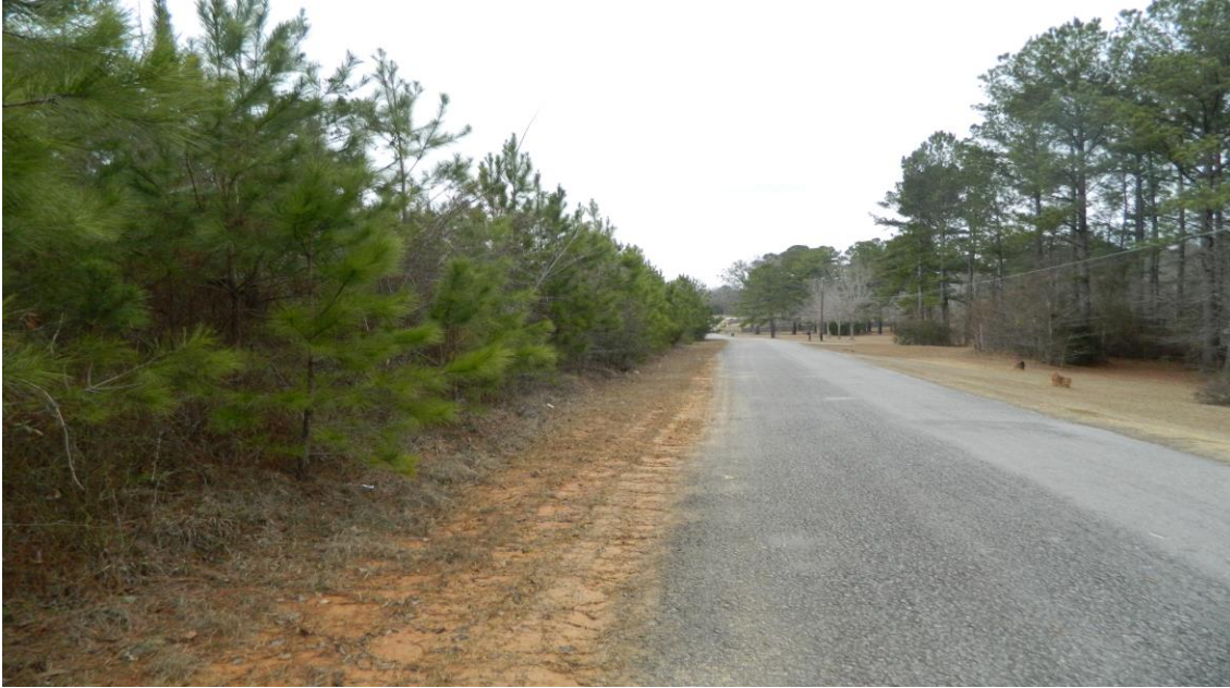
VIEW FACING NORTH ALONG POLLARD ROAD (EASTERN PROPERTY BOUNDARY AT LEFT).
