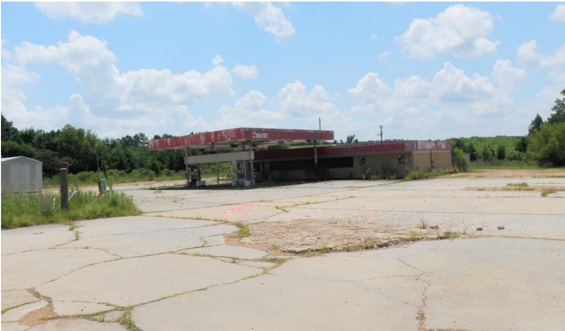
VIEW OF FORMER 25/35 CHEVRON STATION LOCATED ALONG HIGHWAY 25 FRONTAGE ROAD FURTHER TO THE WEST OF THE SUBJECT PROPERTY.
